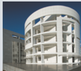
Kirchberg Campus, Weicker building
