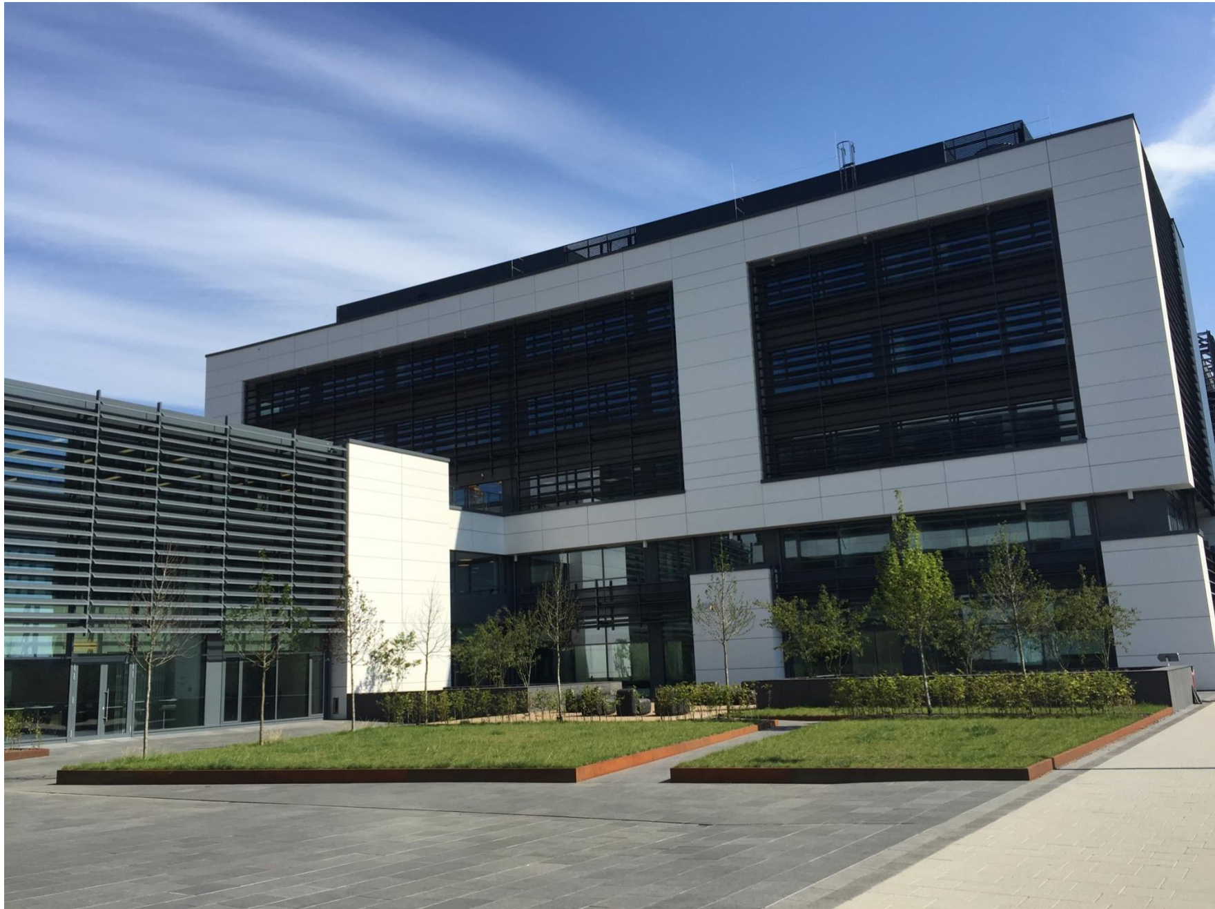
Entrance of the BT2 building without the sculpture – Side view
